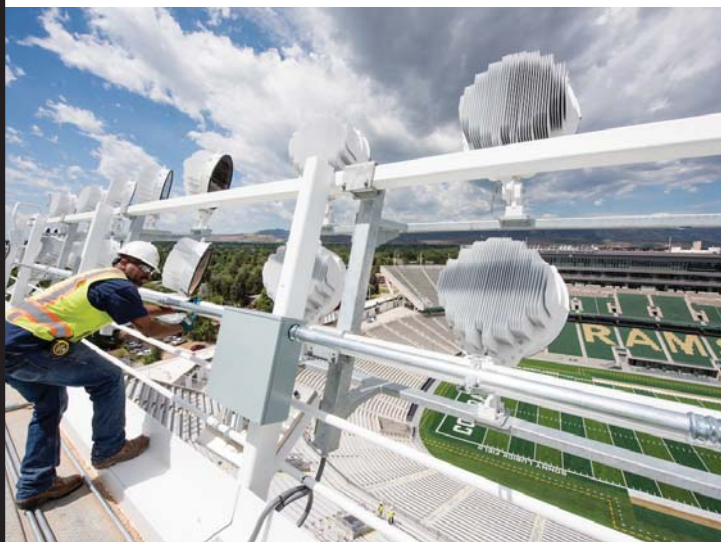
At the new Colorado State University Stadium in Fort Collins, Encore Electric Inc. ( No. 170 ) installed LED sports lights, rather than high-intensity discharge lights. LED lights improved the schedule and the environment. ■
