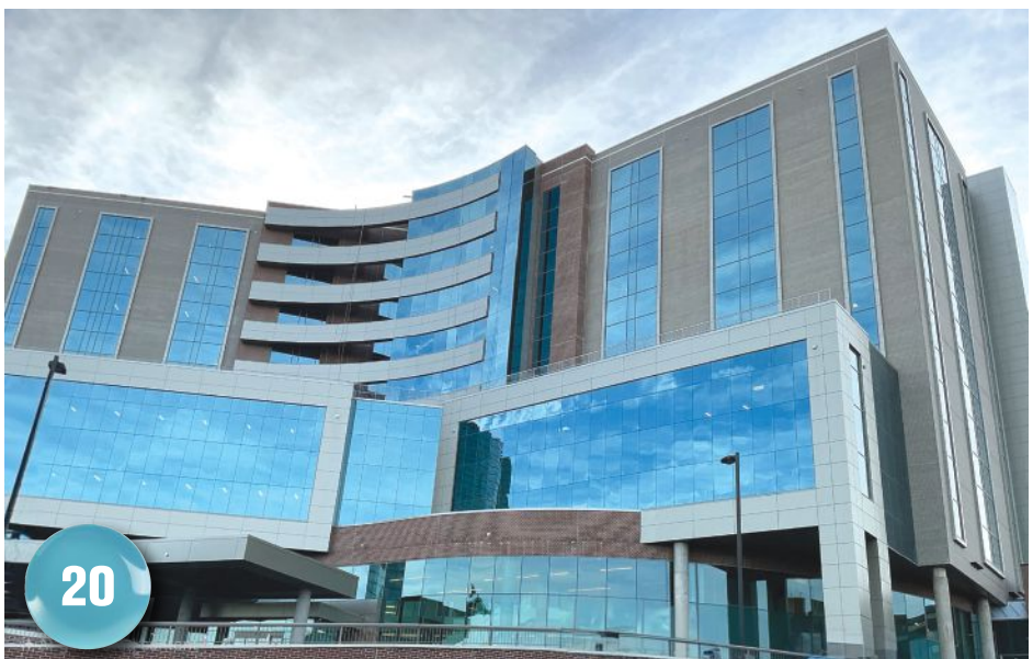
20 SPS Corp. partnered with Robins & Morton/Branch Builds to deliver a $500 million hospital expansion in Roanoke, Virginia. SPS oversaw the fabrication and installation of curtainwall, storefront and ACM panels for the 13-story project.
