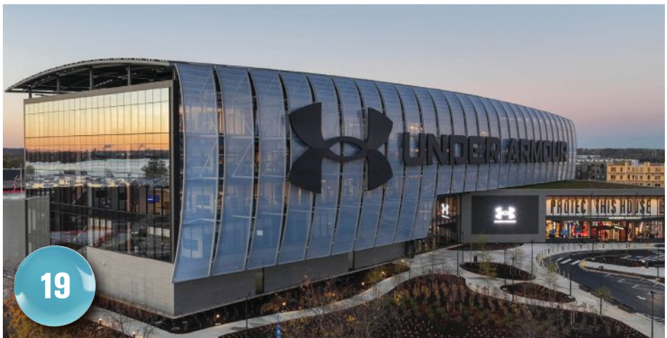
19 Under Armour's new global headquarters in Baltimore features glazing systems installed by Pioneer Cladding & Glazing Systems.
