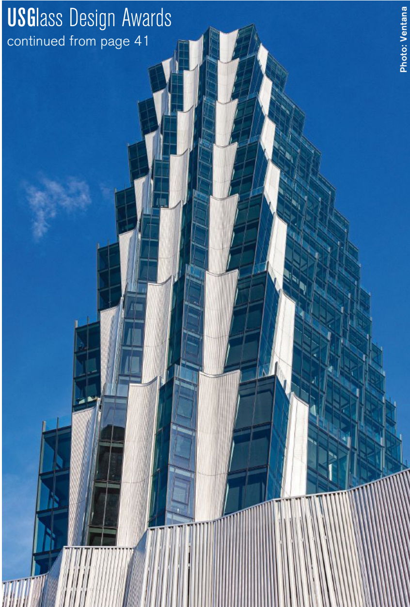
One Hundred Above the Park features an angled glass façade constructed with 135,000 square feet of glass.
